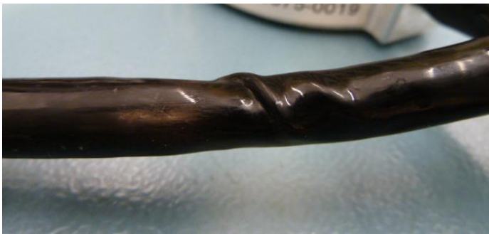
Figure 7: Damaged Motor Cable
