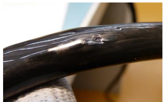
Figure 8: Damaged Motor Cable
